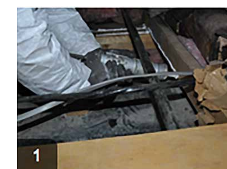
1 Caulk surrounding surfaces before setting cap in place
